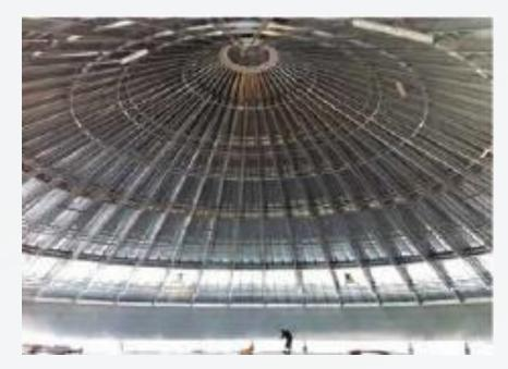
30º degrees roof to optimize storing capacity and Supplied with or without structure depending on the diameter of the silo and roof loads.
