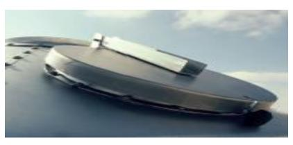
Roof hole allowing the entrance to silo from the roof.
