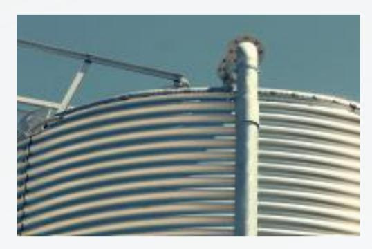
Tube for pneumatic filling, galvanized, diameter 100m, and PVC decompression tube, diameter 160mm. Available mechanic and mechanic-pneumatic.
